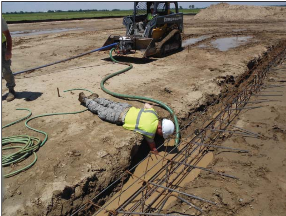
Members of the 477th Civil Engineer Squadron complete repairs on Fletcher Field in Clarksdale, Miss. May 27- June 8. (Courtesy Photo)
